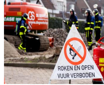
Gas pipe deformations
